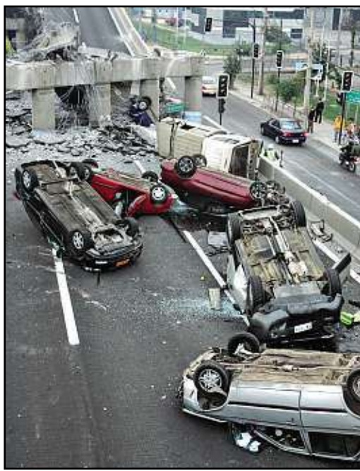
Vehicles are scattered along an elevated highway that collapsed near Santiago on Saturday.
